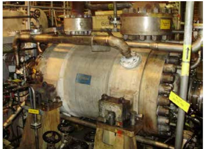
**Figure 3: The intermediate pressure compressor, which was driven by the steam turbine, at the site**
